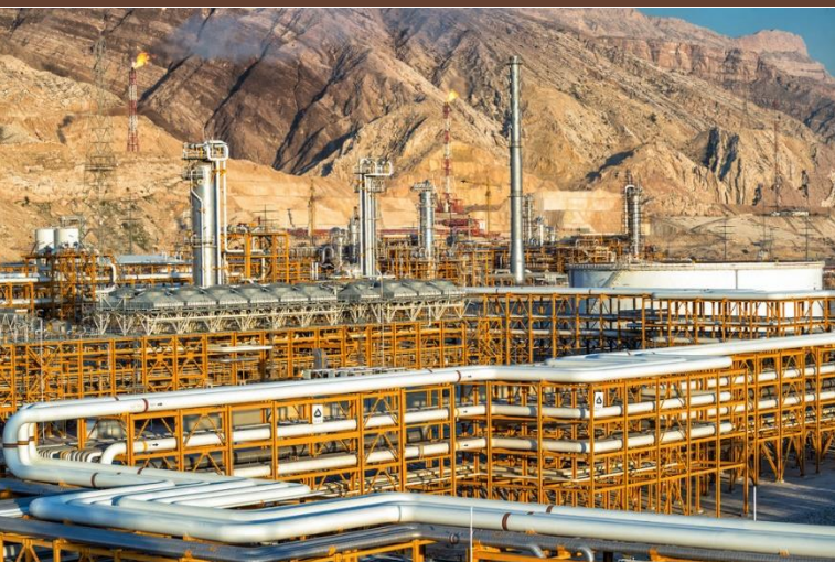
South Pars Gas Field Development, Phases 6,7&8 Refinery, Assaluyeh, Iran
