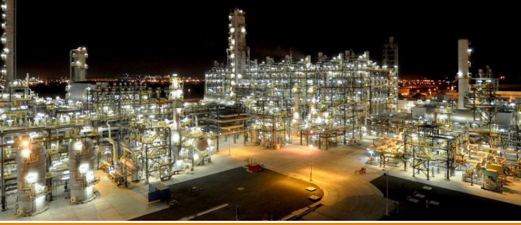
Borouge 2, world's largest ethane cracker, AbuDahbi
